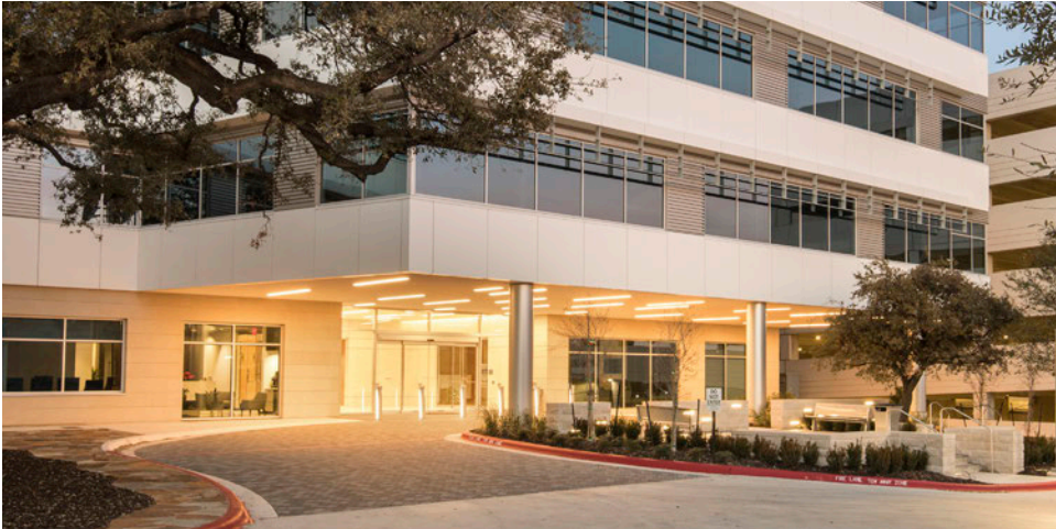
Main Building Entrance
